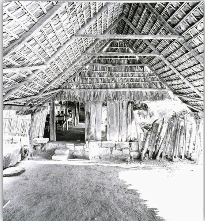
A wood frame and thatched roof structure in Baja California.
