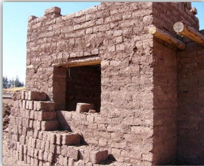
An adobe home with a timber roof structure.
